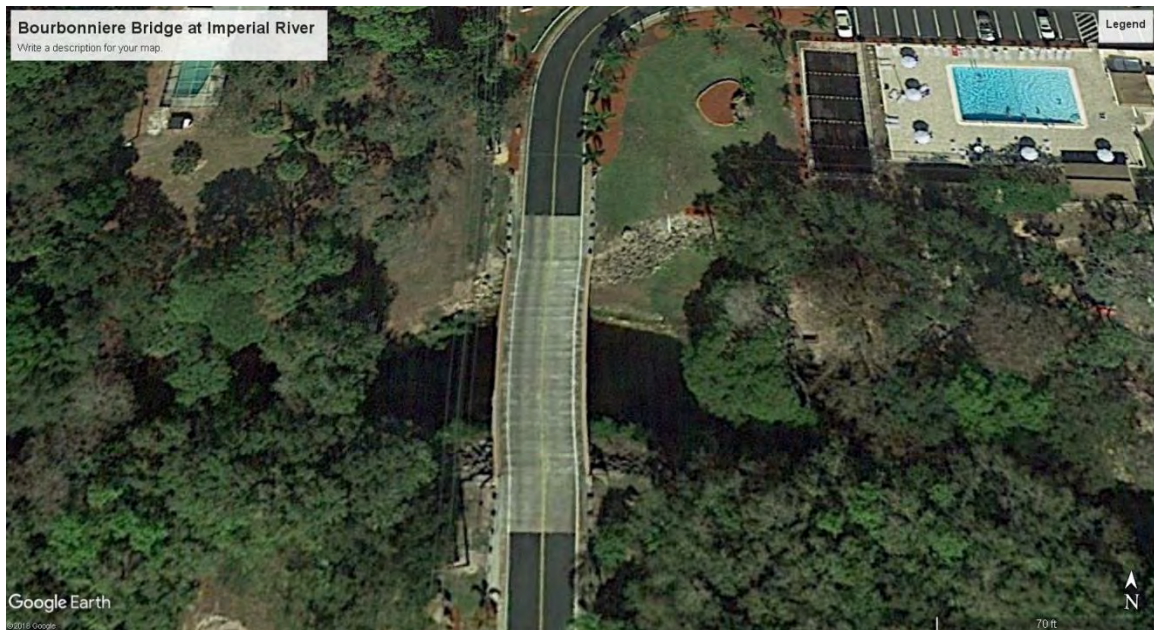
Figure 86: Bourbonniere Bridge crossing of the Imperial River
