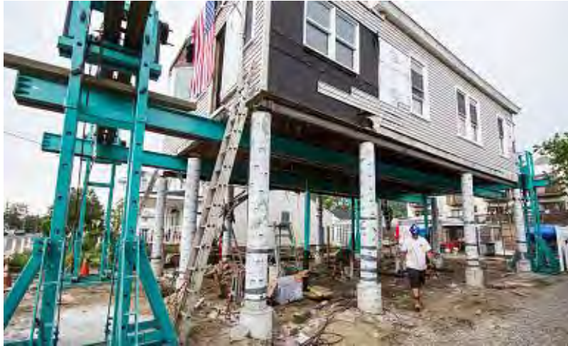
Figure 112: Elevating a House Out of a Floodplain in Louisiana
