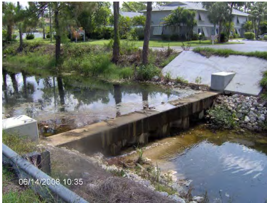
Figure 73. San Carlos Estates southernmost weir. Note: flow from erosion. Source: 2008, Exceptional Engineering, Inc.
