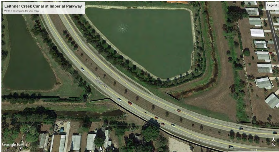
Figure 90: Leitner Creek Canal culvert crossing at Imperial Parkway
