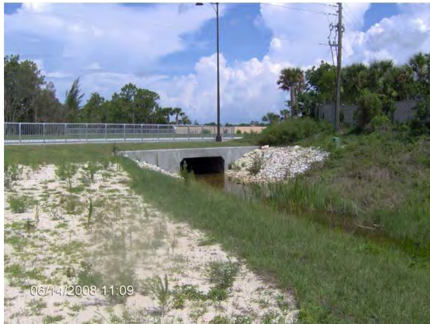
Figure 54: Box Culvert at Three Oaks Parkway Extension east side Source: 2008, Exceptional Engineering, Inc.
