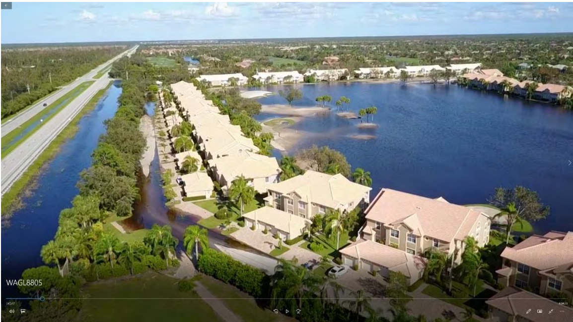
Figure 38: Flooded Areas City of Bonita Springs at Worthington and Bonita Beach Road East. Source: City of Bonita Springs
