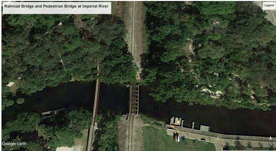
Figure 96: Railroad Bridge and Pedestrian Bridge Crossings of the Imperial River
