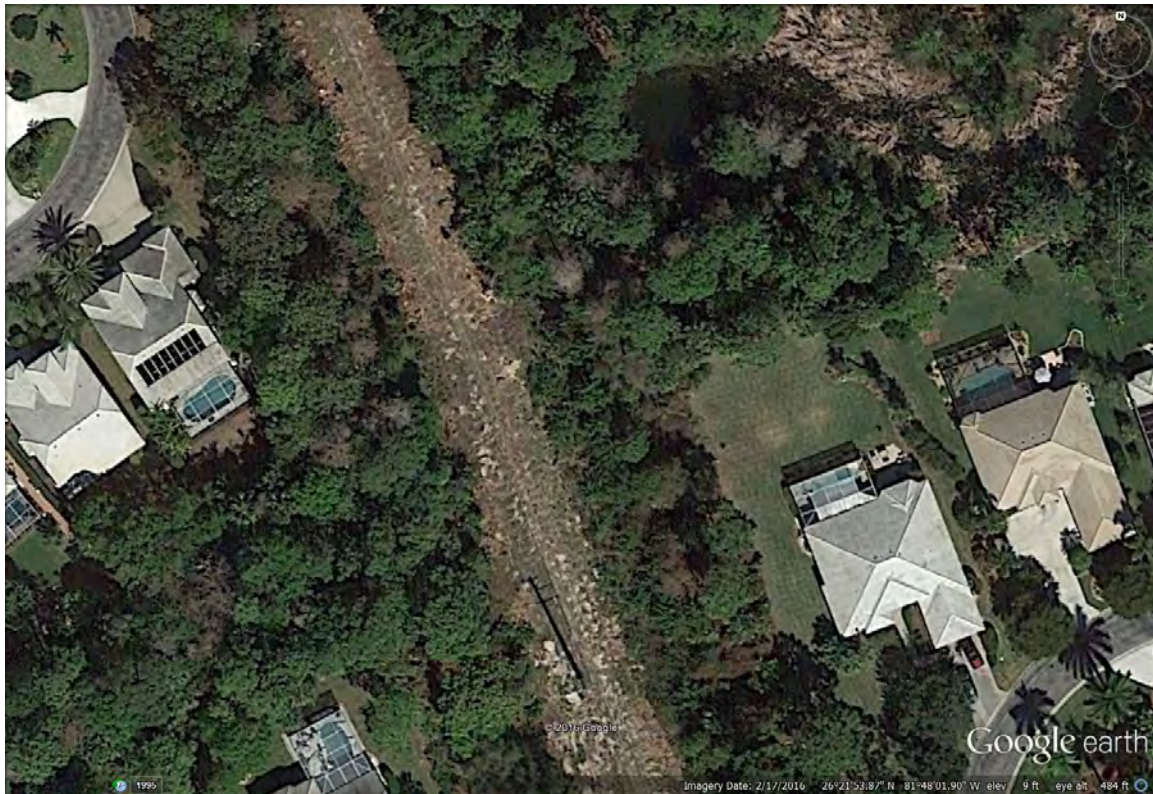
Figure 60: 48” RCP at FPL easement Source: 2008, Exceptional Engineering
