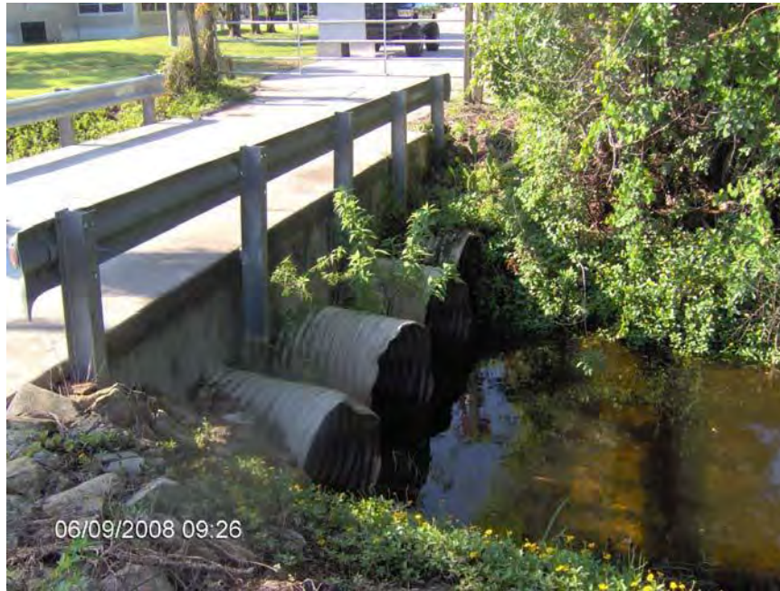
Pic 14. Imperial Harbor CMP pipe crossing. Figure 72: Imperial Harbor CMP pipe crossing. Source 2008, Exceptional Engineering, Inc.
