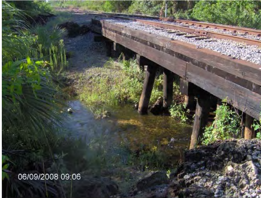
Pic 12. Seminole Gulf Railroad Crossing
