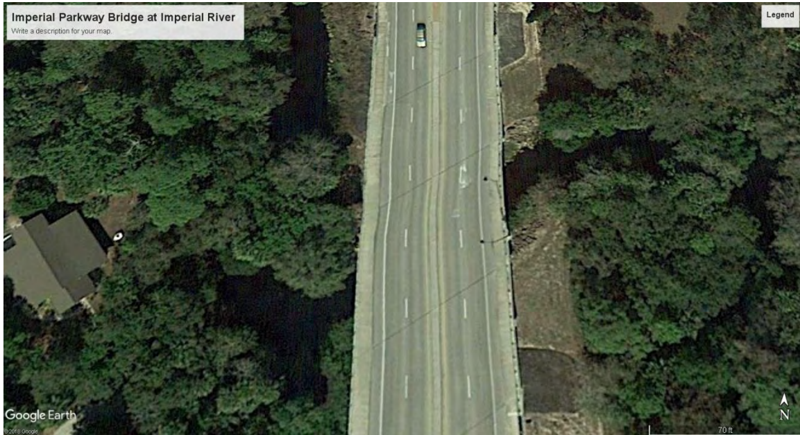
Figure 87: Imperial Parkway Bridge crossing of the Imperial River
