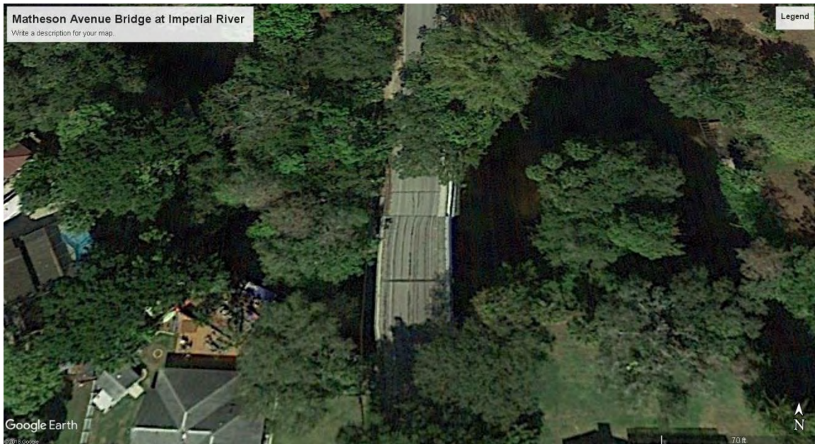
Figure 88: Matheson Avenue Bridge crossing of the Imperial River
