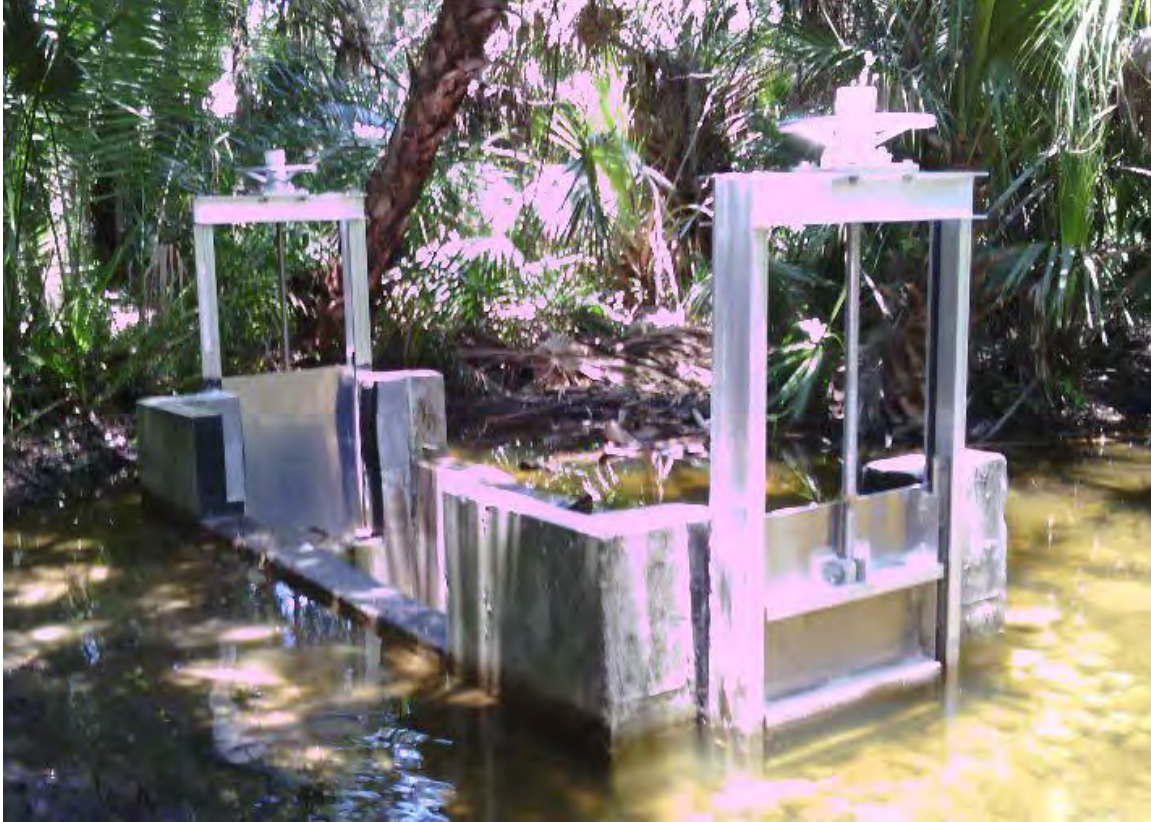
Figure 113: Emergency Sluice Gate at Pelican Landing
